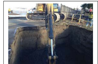
Excavation for final light pole at Cargo 6
